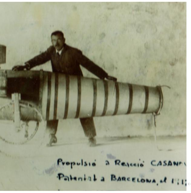
Ramon Casanova and the pulsejet engine he constructed and patented in 1917 Photo: Jcrbmc, 1916 | Wikimedia Commons
