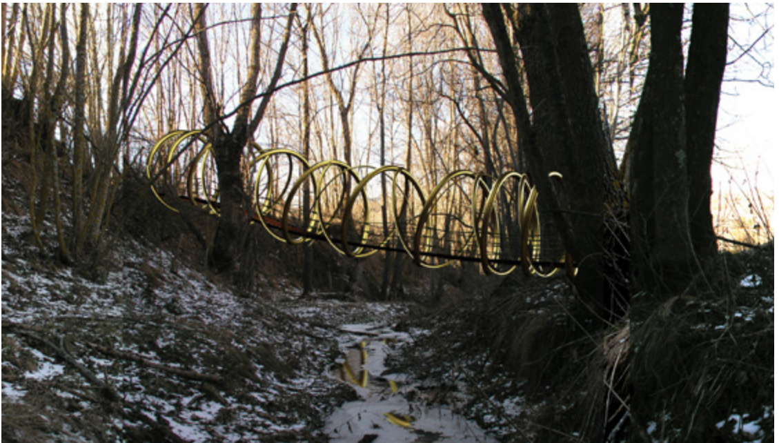
Fig 8. Footbridge for the Pyrenees. Dennis Dollens and Ignasi Pérez Arnal. Based on three intersecting helicoids whose data was captured from flying seedpods; the bridge strives to fit onto the site with minimal sculptural presence and no destruction to the land or existing trees.
